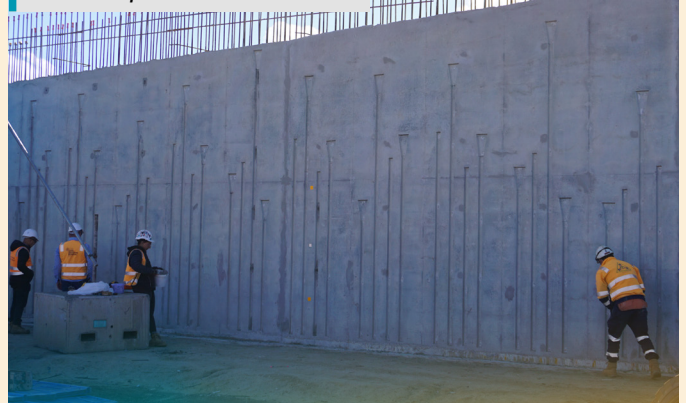
Crews working on the abutment wall at Hopkins Road.
