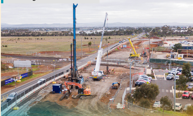
Piling rigs at Ferris Road for road bridge foundation works.
